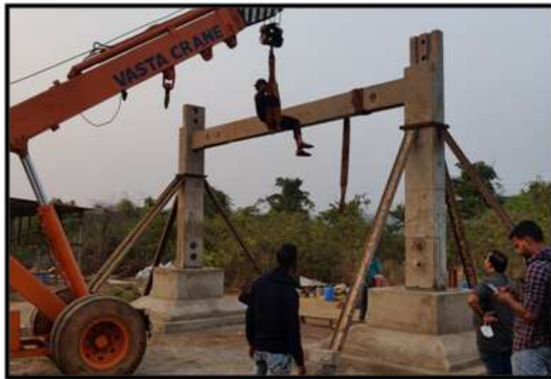
FIGURE 22: ASSEMBLY OF FRAME IN PROGRESS
