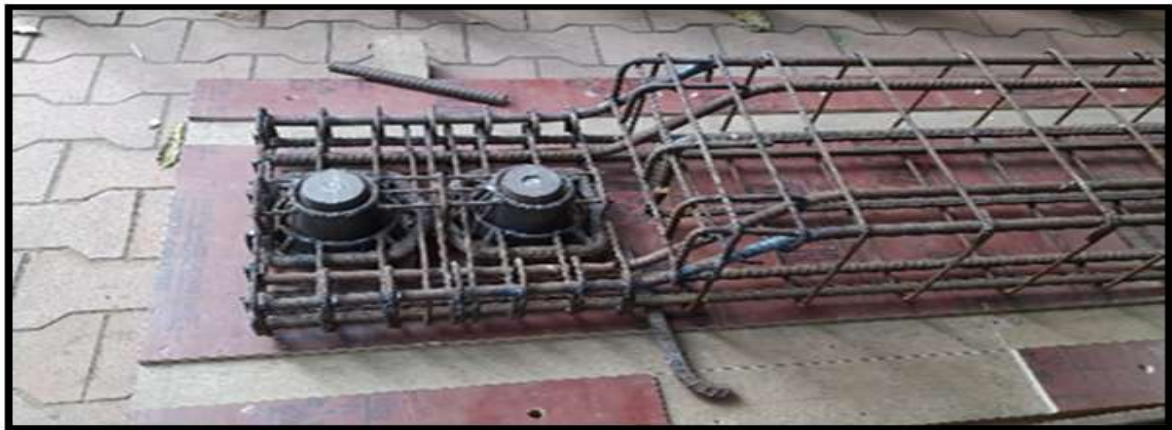
FIGURE 17: COLUMN CONNECTION CAGE
