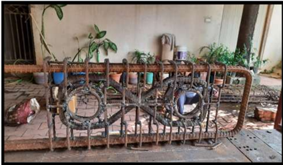
FIGURE16: CONNECTION CAGE WITH INFINITYRING.
