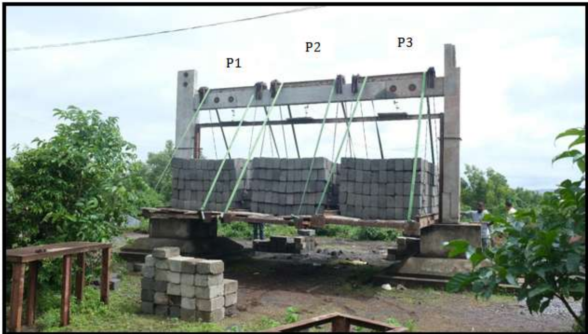
FIGURE 55: FULLY LOADED SUSPENDED PLATFORM.
