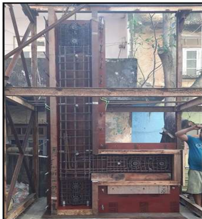
FIGURE 18: REINFORCEMENT IN WOODEN SHUTTERING.
