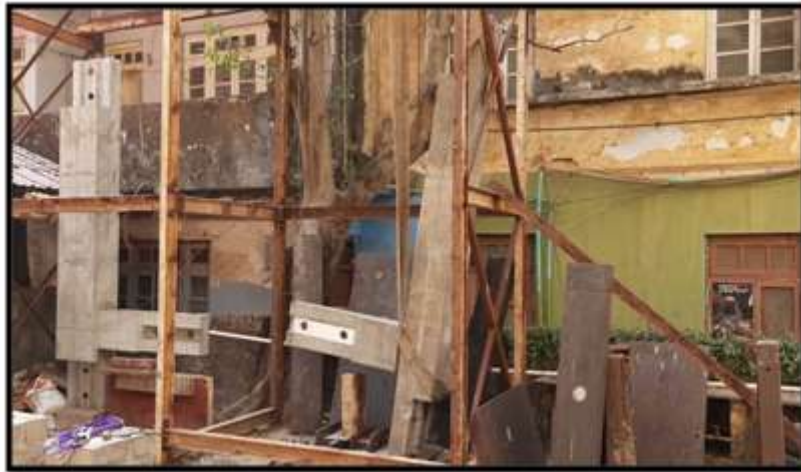
FIGURE 21: COLUMNS AFTER DE-SHUTTERING, READY FOR TRANSPORTATION
