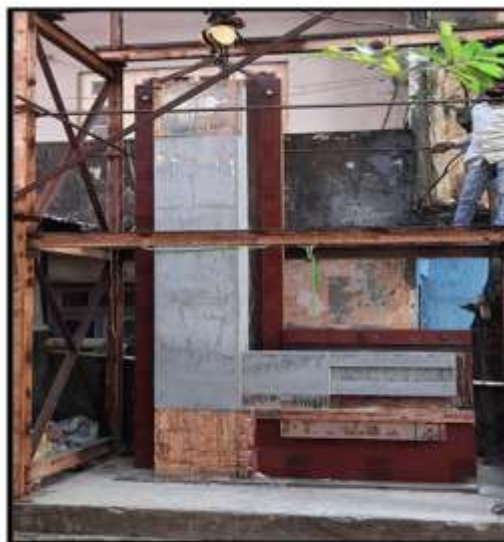
FIGURE 20: COLUMN AFTER DE-SHUTTERING.
