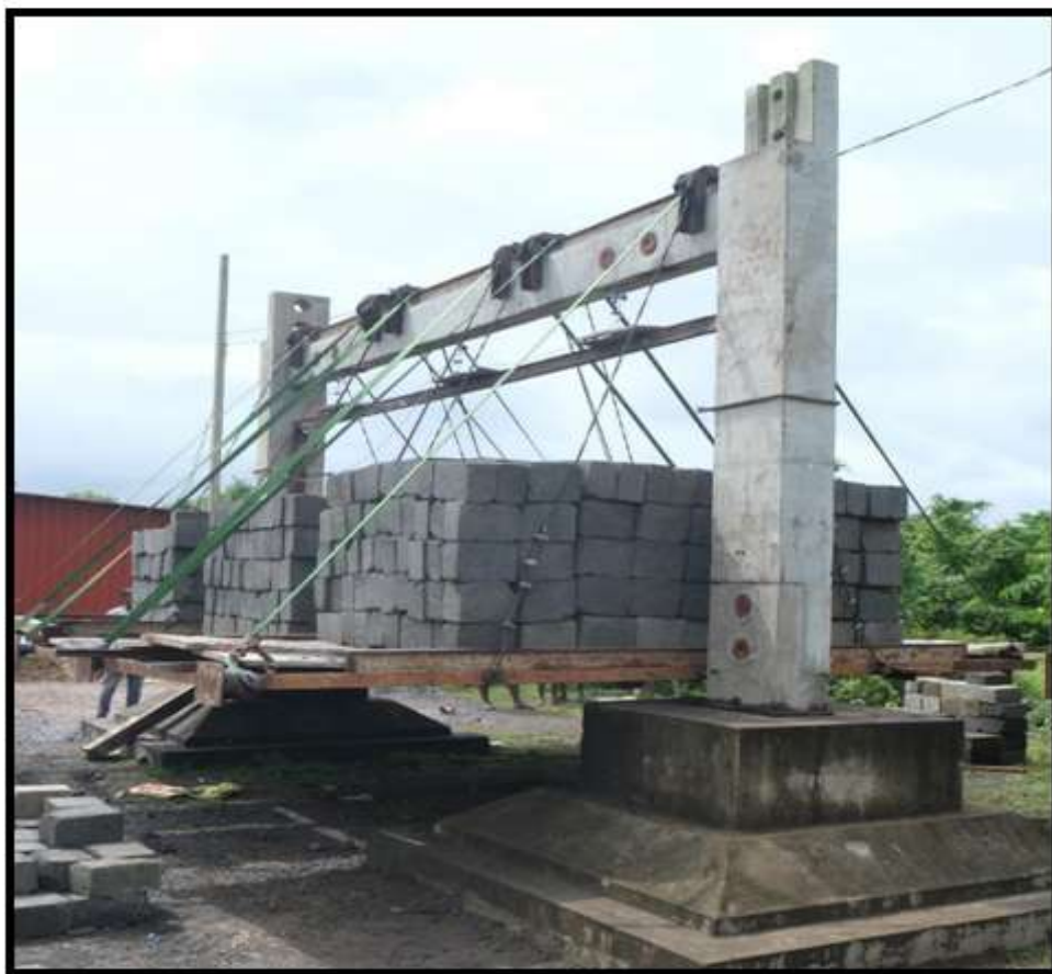
FIGURE 56: FULLY LOADED SUSPENDED PLATFORM. – SIDE VIEW
